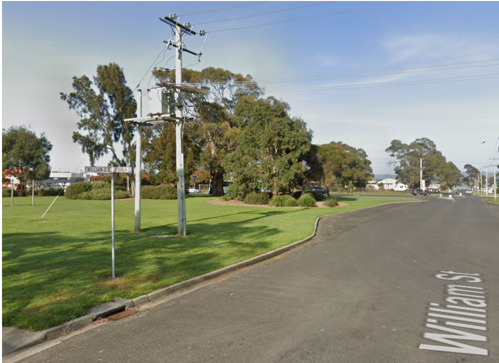
Authority Pole Mounted Sub-Station on William Street
