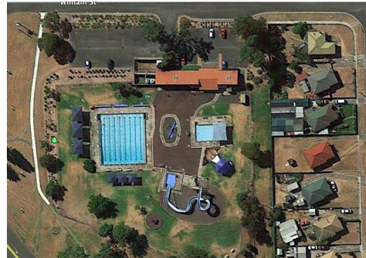
Figure 2 Aerial view of George Town Swimming Pool
