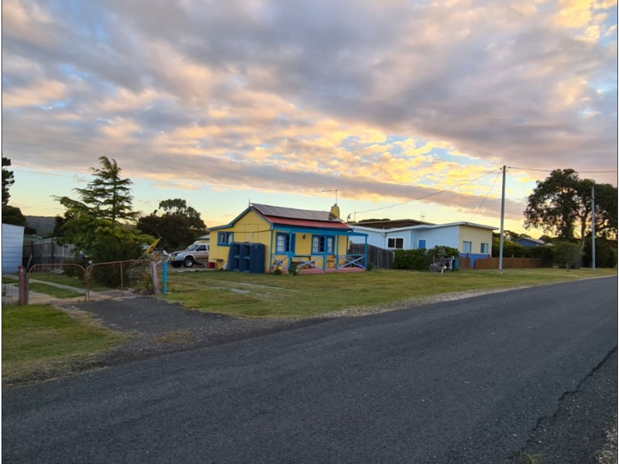
Figure 4 – View of the existing dwelling at 4 Davies Street, looking south-west.
