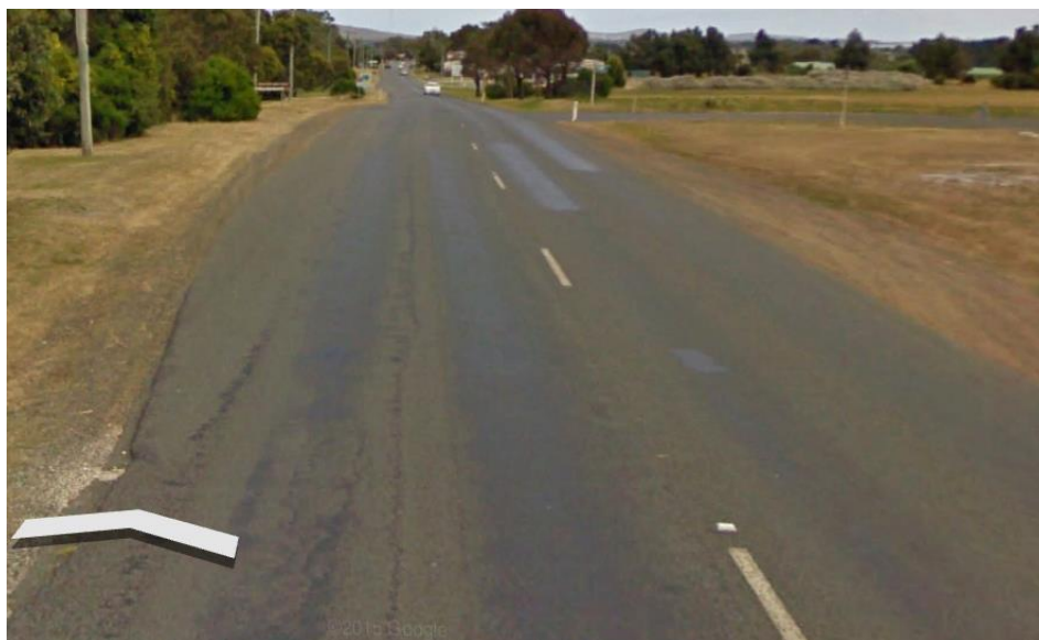
Photograph 6.9C – BAR turn treatment on the East Tamar Highway
