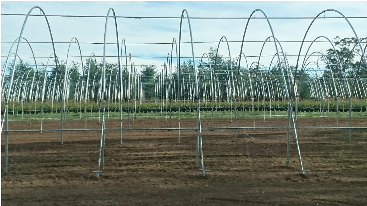
Figure 6 Tunnel structure framework and footings
