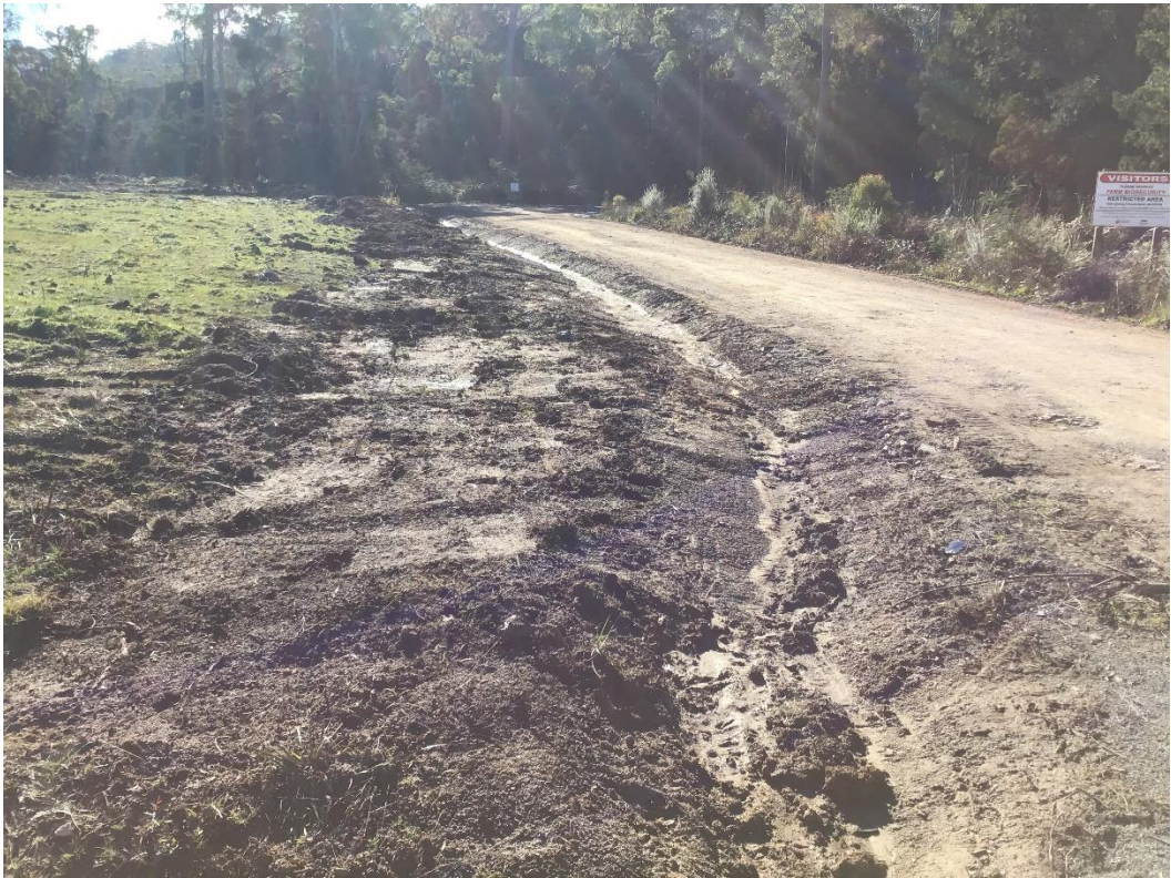
Figure 8 Current drain located at the southern end of the development area which directs runoff from Hillwood Road into the Macquarie Rivulet
