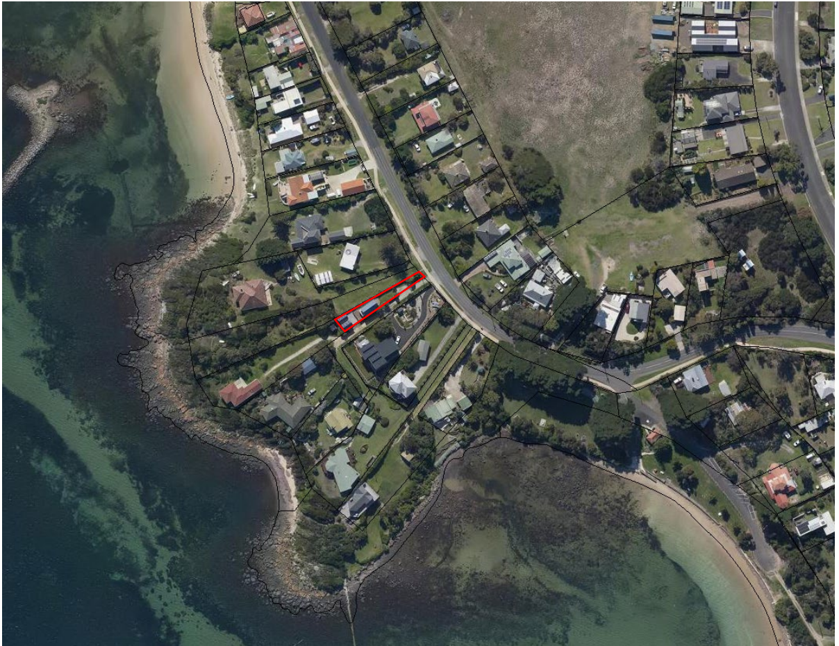
Figure 2: Aerial view of Cordell Point, showing the subject site outlined in red, and adjoining lots.
