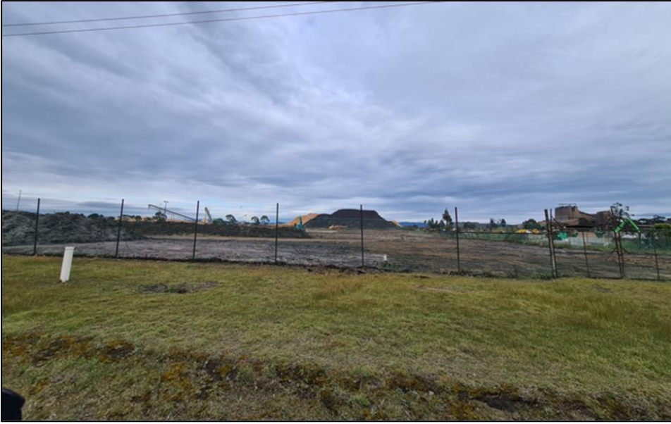
Figure 6: Subject property, looking south-west from Norfolk Street.
