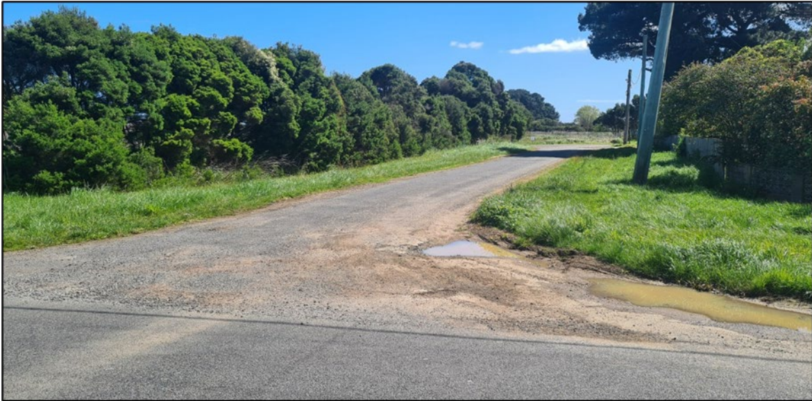
Figure 7: Site Photos –Arthur Street looking north into Elizabeth Street Road Reserve
