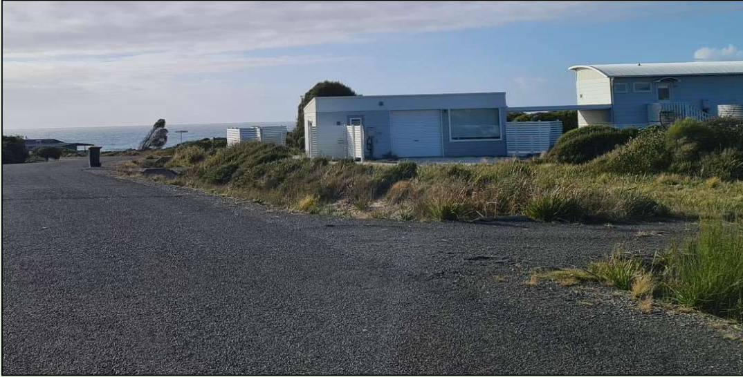
Figure 9: Existing outbuilding at 52 Seascapes Drive.
