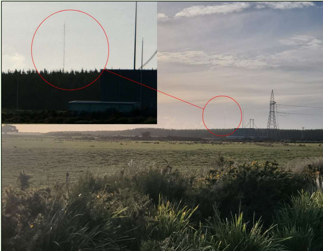
Figure 6: Existing met. mast showing the mitigating impacts of separation.
