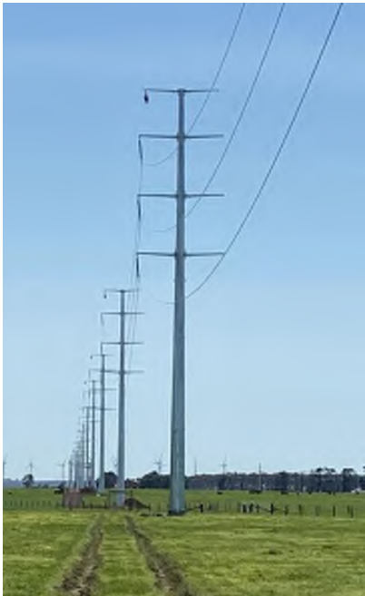
Figure 21. Typical double circuit pole transmission line
