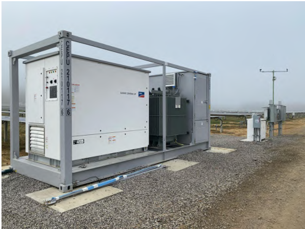
Figure 17. Power conversion unit (Source:SMA)
