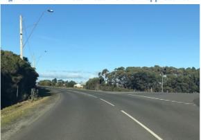
The Low Head Road South bound lane should be widened to fit a Basic Right turn facility.
