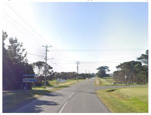
The Low Head Road North bound lane should be widened to fit a Basic Right turn facility.
