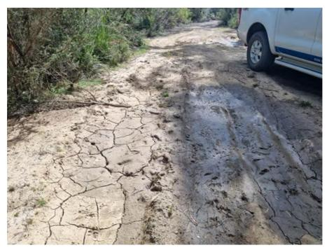
Photo 12. Desiccation cracking in brown, low to medium plasticity clay on access road.
