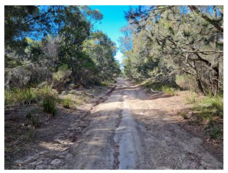
Photo 3. Silty sand with sandstone gravel (possible colluvium derived from Permian-aged sandstone), road washed out due to surface runoff, looking south.
