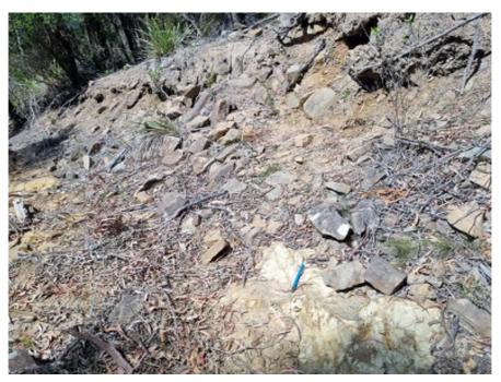
Photo 17. Highly weathered dolerite bedrock overlain by ~1.2m of colluvium, road cutting has been undercut by erosion, looking southwest.
