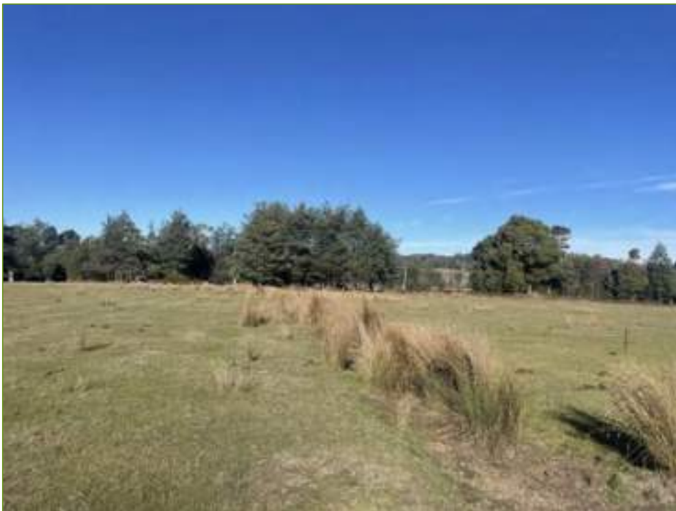
Figure 23 The western boundary on the subject property, facing south. Boundary fencing between the subject property and the adjacent title TR: 52896/3 is in disrepair. Taken at site assessment 29/5/2025.
