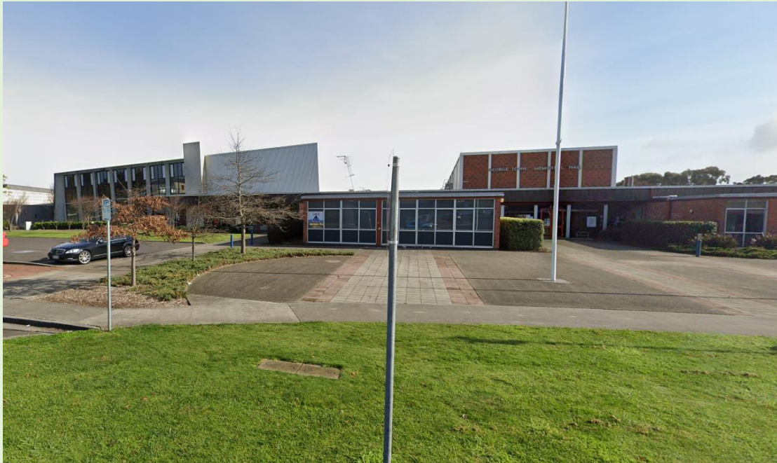
Figure 6: Memorial Hall (11m)
