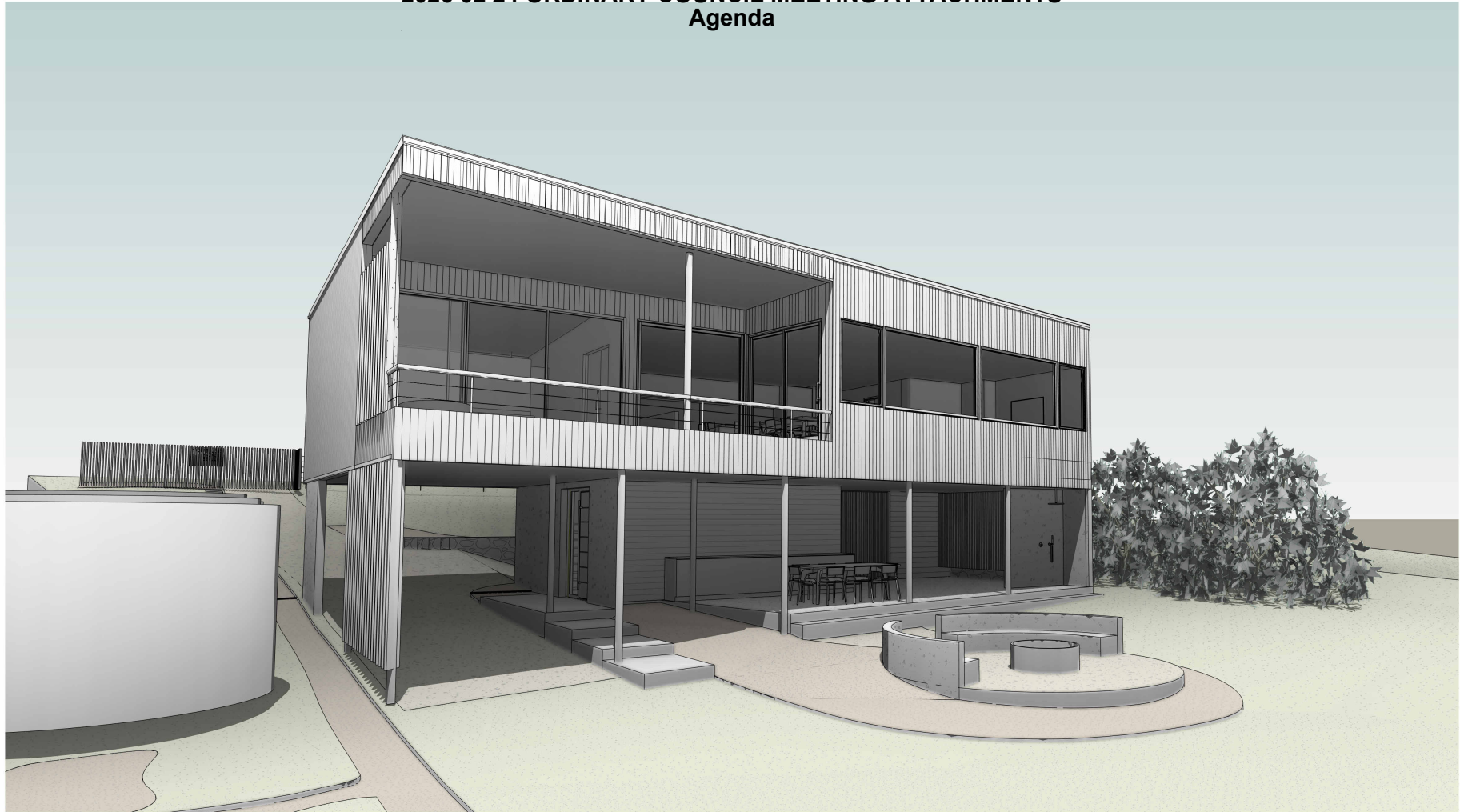
1 OCEAN FACING FACADE
