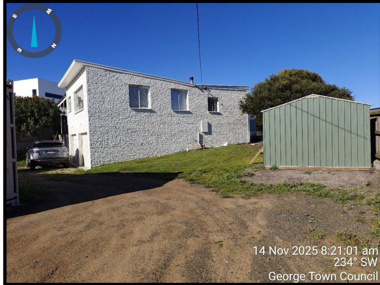
Plate 1: Existing dwelling and shed looking to the southwest.
